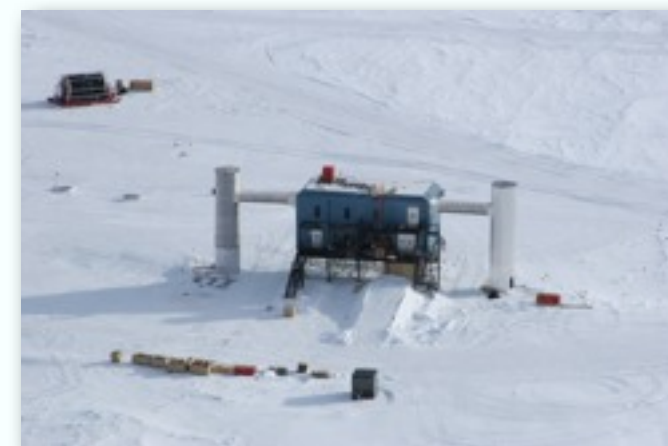
IceCube Lab (ICL) central computing facility
